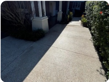
02 The same driveway, after Cleaned, not resurfaced.
