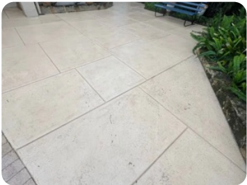
04 The same courtyard, after Clean, and ready to seal.
